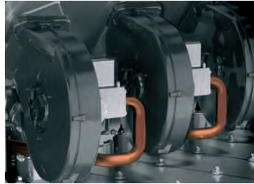
Pre-mix burners with individual fans and gas valves.
