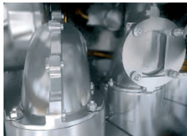
Integrated non-return flue valves.
